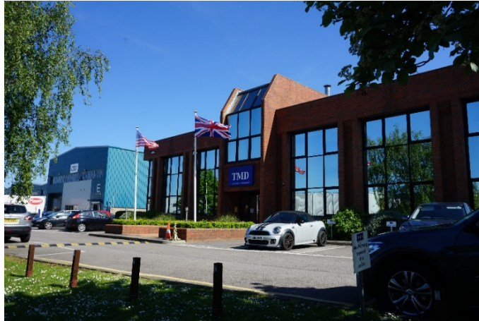
TMD's headquarters design and manufacturing facility in West London, UK.
